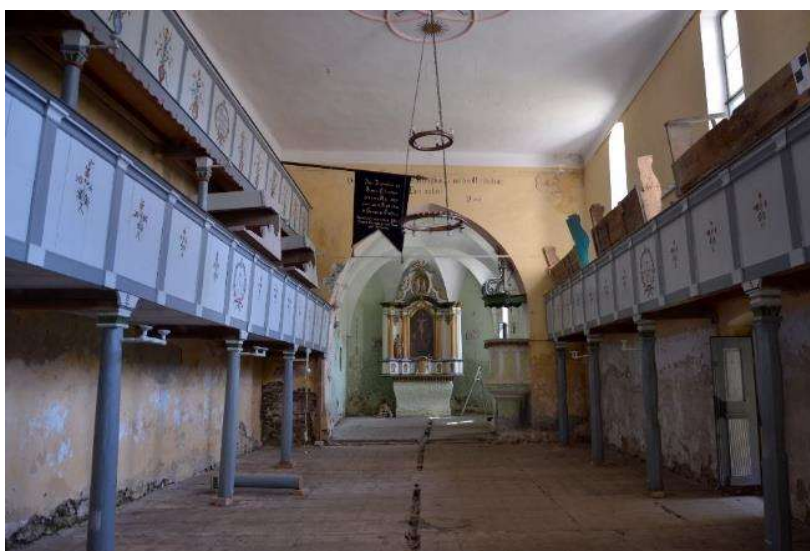
Fig. 08 a-b. Church's interior (left) in 2014 and (right) in 2019 after the after removal the floor and the wooden elements affected from the fungus boletus destructor
